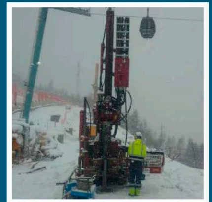
Boreholes with Sonic technology
