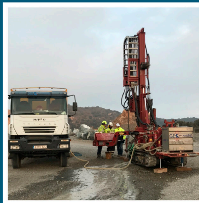
Drilling with Sonic Drilling system
