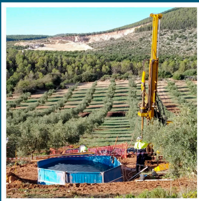
Drilling with Wire-Line system
